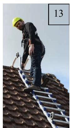
Push the wheels upwards beyond the roof ridge and then turn the ladder (9) over, so that the ridge hook lies against the other slope of the roof (10-11).
